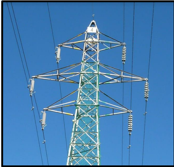
Pic 4: 66KV ACSR® line in Japan
