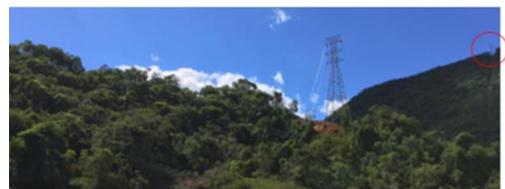
Pic 5: 1087m long span (300m elevation difference)
